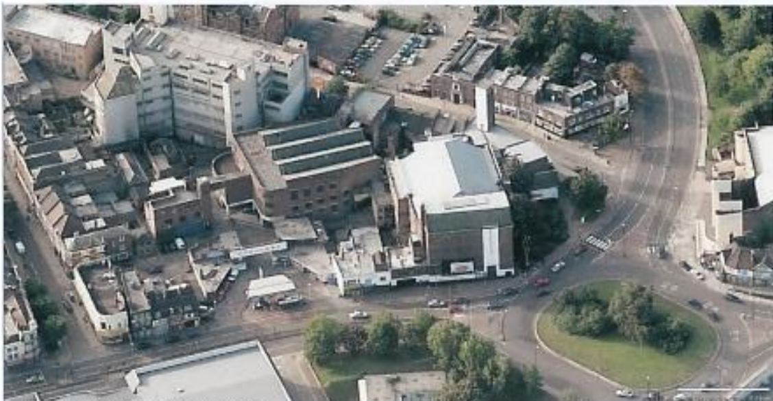
Woolwich High Street Elevation
